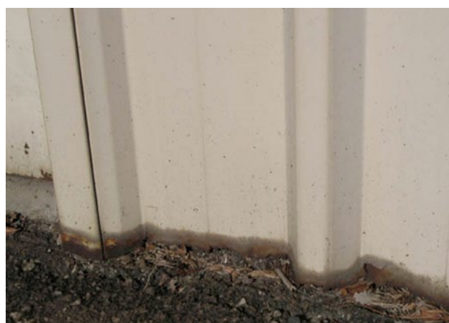
Figure 2. Corrosion due to inappropriate wall design
