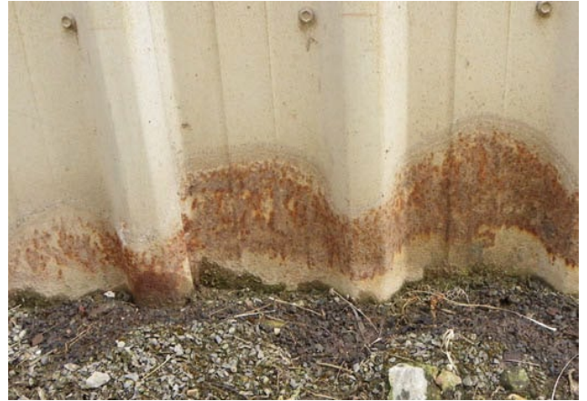
Figure 3. Corrosion due to immersion in soil
